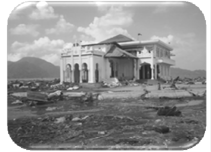
Masjid in Banda Aceh after Tsunami
